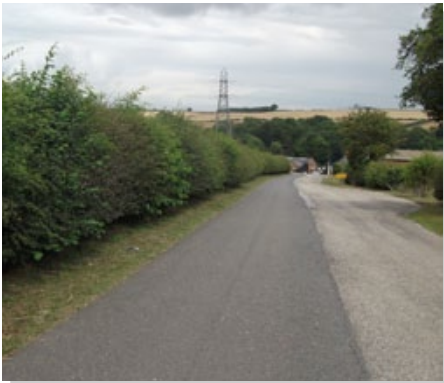
Access road to existing water treatment works
