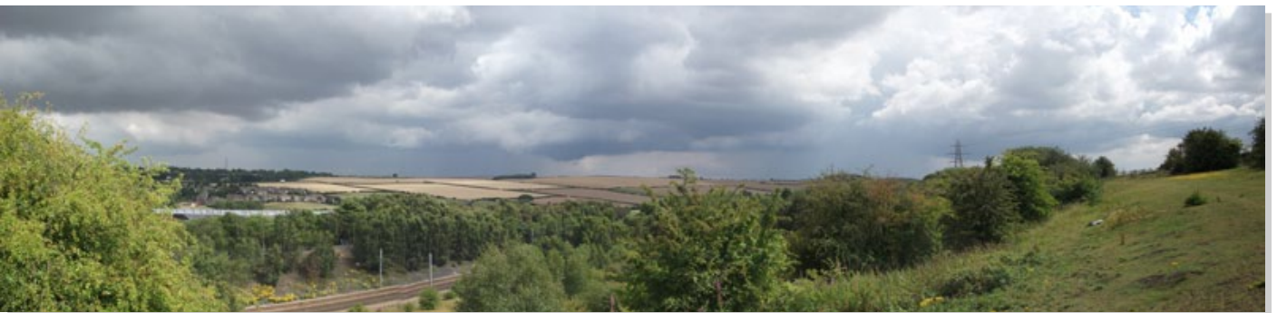
View south east across the rail and river corridors
