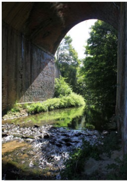
River Witham below the existing rail viaduct
