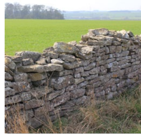
Parish boundary wall (in the ownership of the adjoining land owner to the south)
